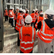
JHS' students see the insides of Pike as construction continues
